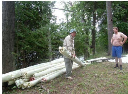
11. Master mat construction technician Jim with a pile of mats. Diver Mike is here to pick up a load.
