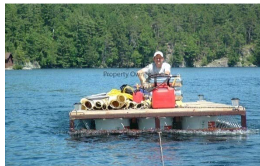
5. The work float was towed to the staging area. It worked real well for a first time boat designer/builder.
