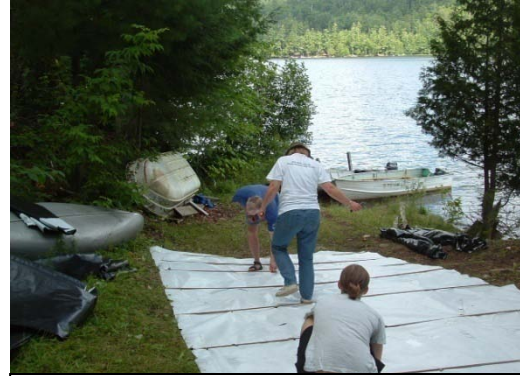
10. The mat assembly crew finishing installation of zip ties used to hold ballast to the plastic tarp (mat). Next step is to roll them up. Not a lot of extra room on this sloped work area, but better than no site.
