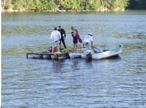
13. Working on the western (smaller) basin of the lake without the benefit of the pontoon boat. This is the first patch mats were laid on.
