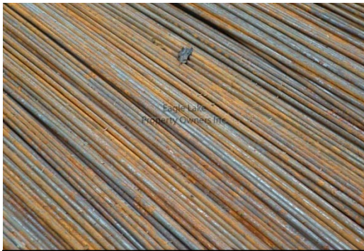
8. Steel bars and more steel bars. Pictured here, 3500lbs of 10 foot ballast hand carried from the road approximately 200 feet to the mat assembly area. In all, more than 11,000 lbs were used.
