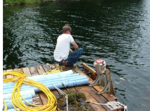
16. Setting anchor and getting ready to deploy more mats. One of the 4-150' air lines coiled up. Keeping them untangled as divers swam around was a continuous and daily chore.
