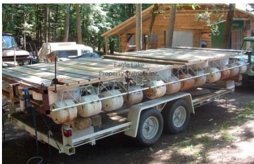
2. Work float construction almost complete.
