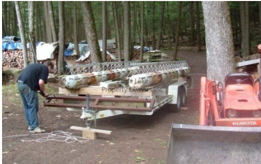
1. Constructing the work float.
