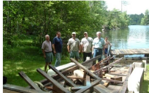
4. The launch crew lifted the float off the trailer and set it on saw horses. The trailer was removed and the float was then set down in the water.
